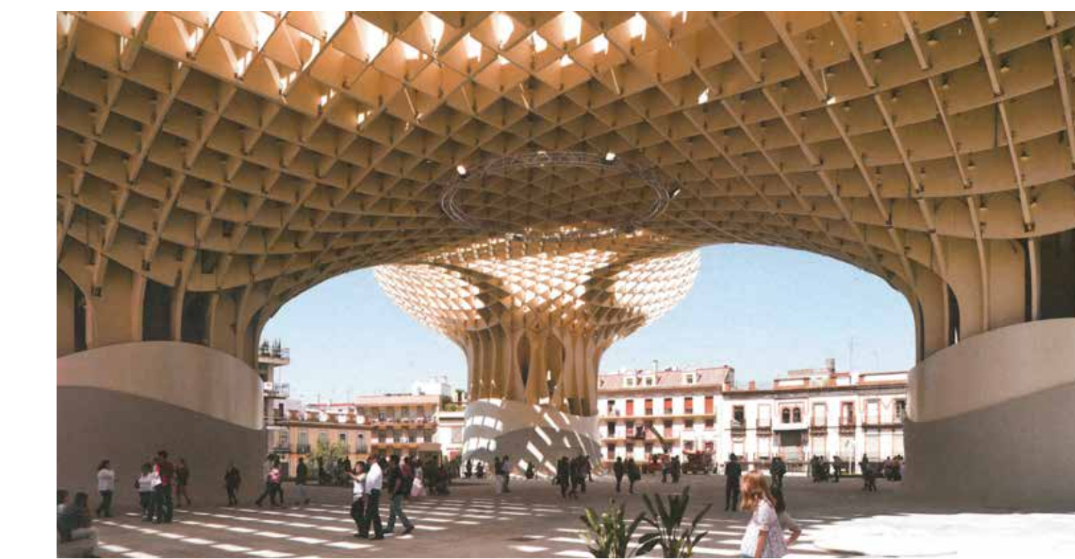
Public plaza with canopy, Seville, Spain.
