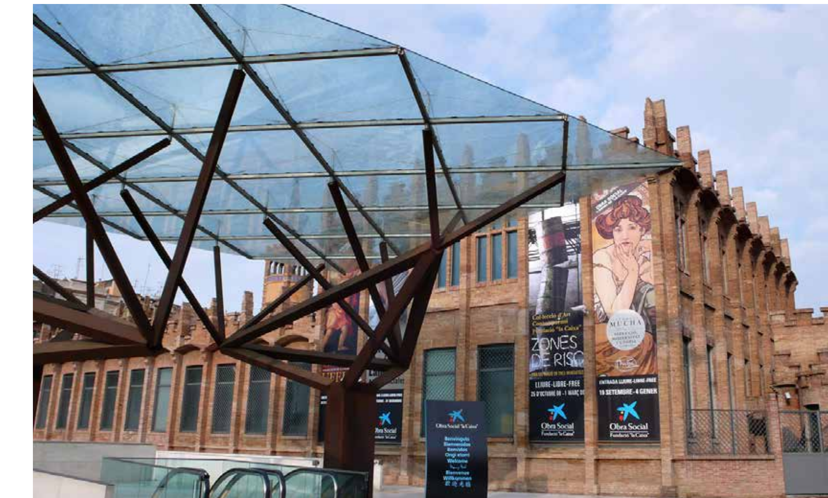
Glass canopy at Metro plaza, Barcelona, Spain.
