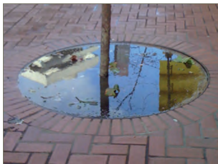
Soil drainage issues
