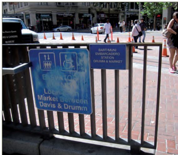
Muni underground signage retrofitted to portal railings are vandal prone.
