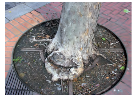
Grate frame cutting root flare
