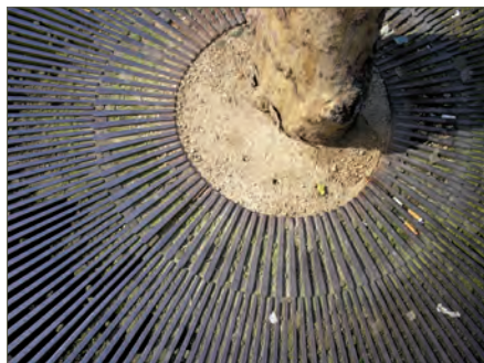
Debris clogged grates
