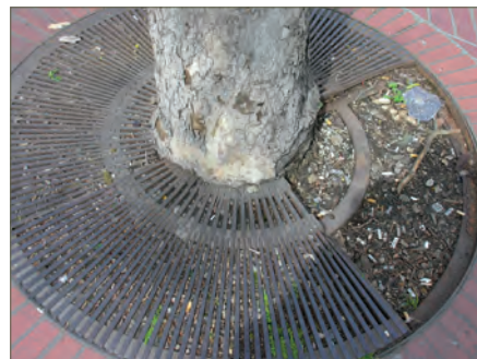
Tree out-growing grate condition
