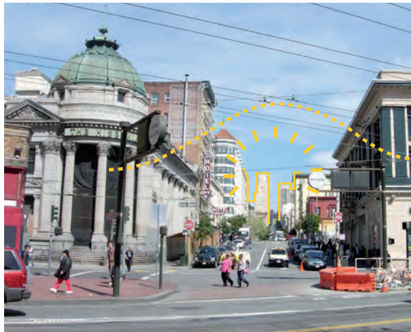
Market Street @ Jones - north-east view
