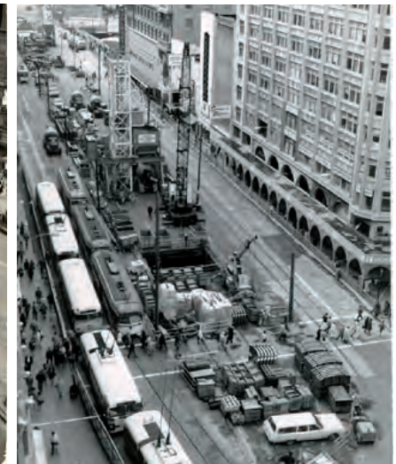
BART construction 1970 4th @ Market
