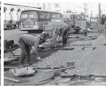
Paving of Market Street sidewalks
