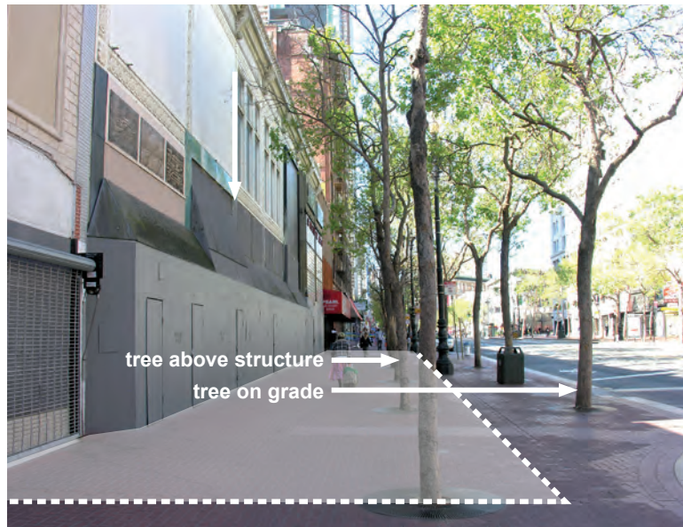
Subsurface condition might compromise soil volume and tree health
