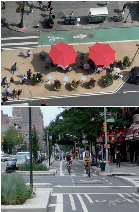
'Copenhagen Style' bicycle track separates bicycles from pedestrians and car traffic. New York City
